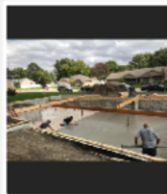
Building Trades students pouring a floor at the homesite.
